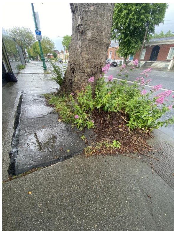
Photo 4: Views of pavement lift on footpath.
