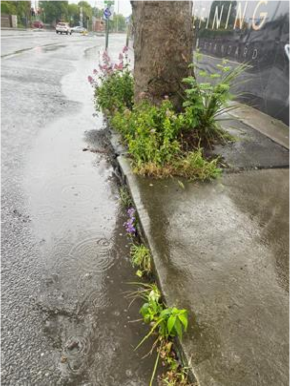
Photo 8: Views of distortion to kerb adjacent to road.
